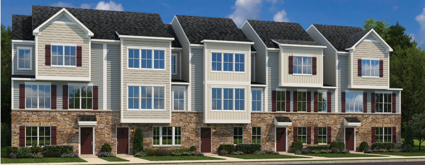
BASEMENT LEVEL ENTRY W/ REAR GARAGE
