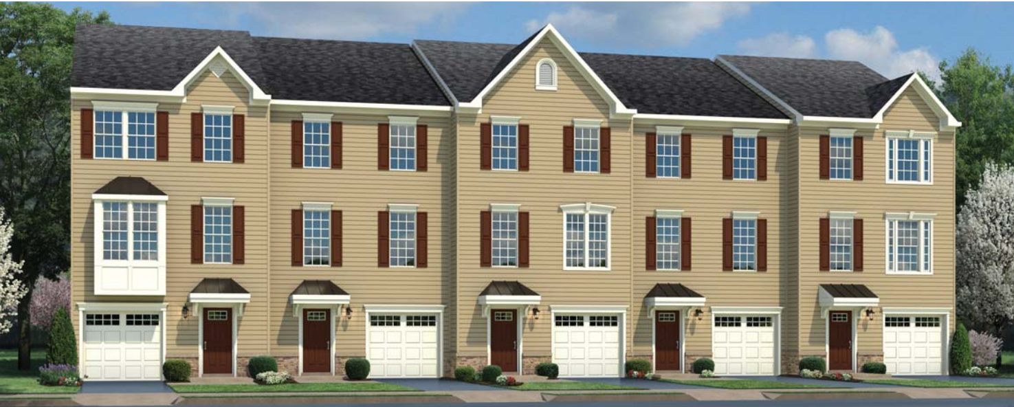
BASEMENT LEVEL ENTRY
