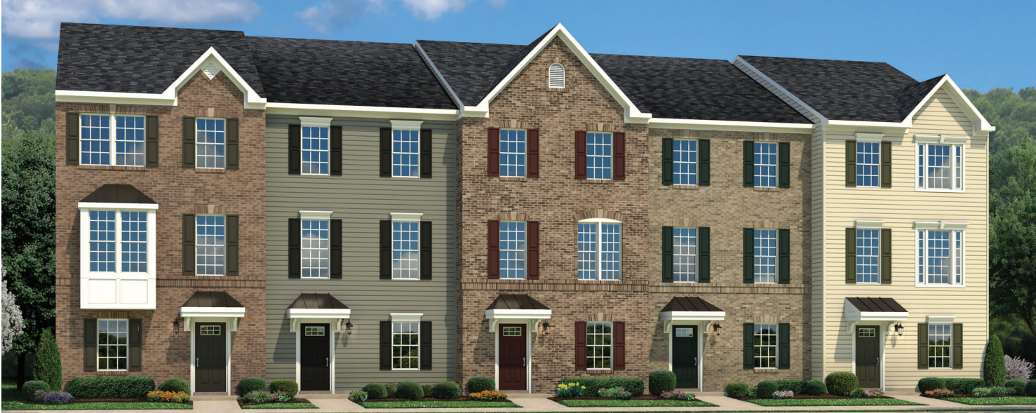
LOWER LEVEL ENTRY
