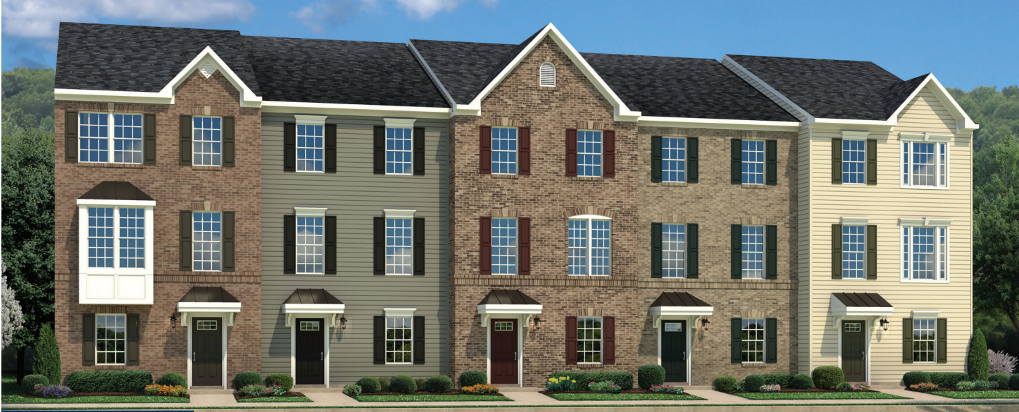
LOWER LEVEL ENTRY
