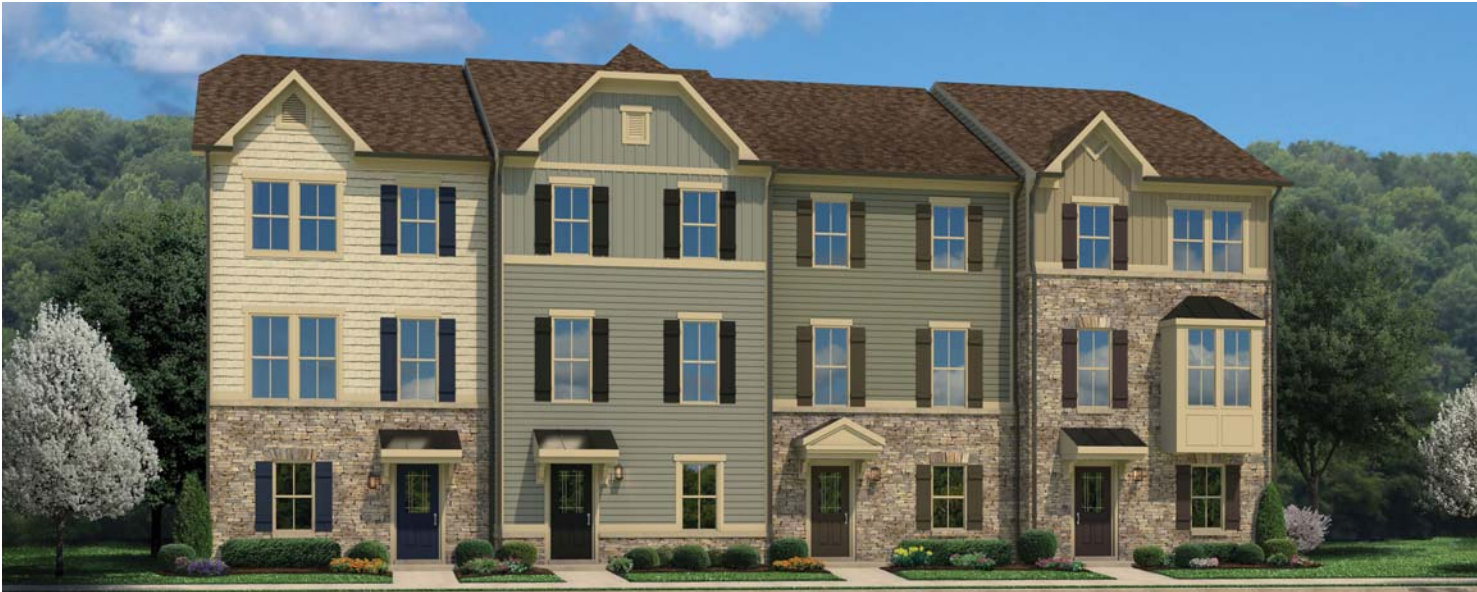
BASEMENT LEVEL ENTRY
