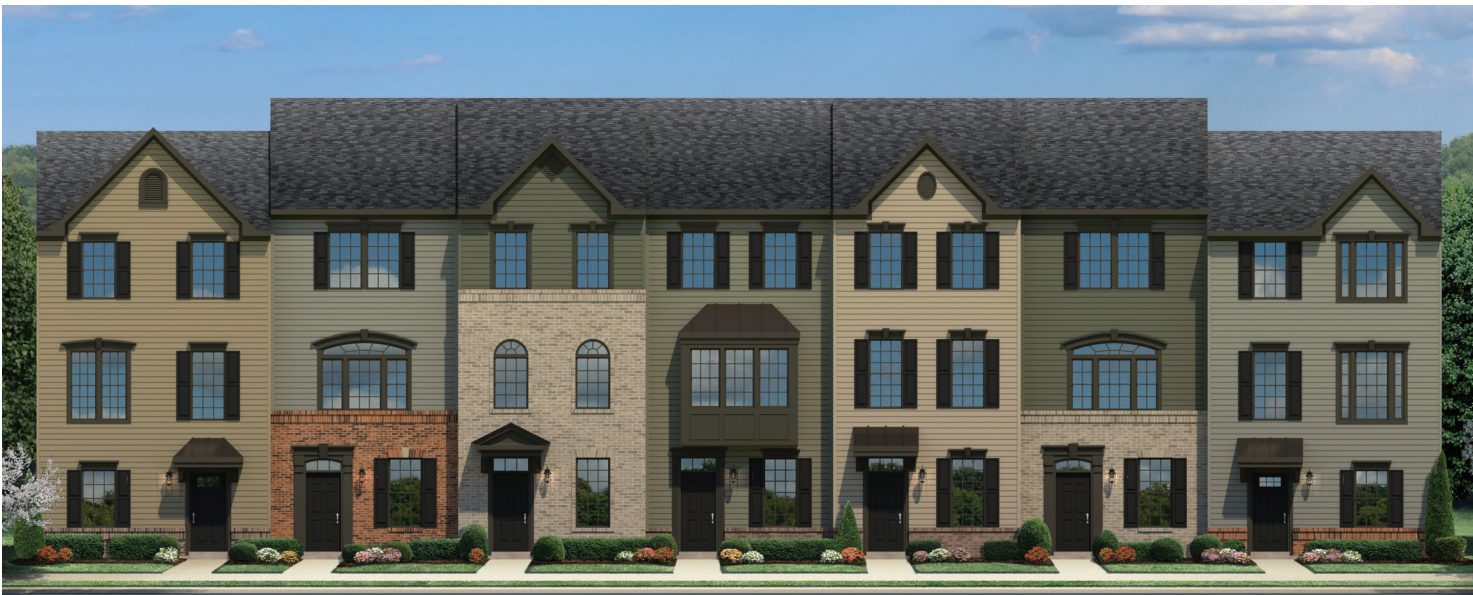
LOWER LEVEL ENTRY
