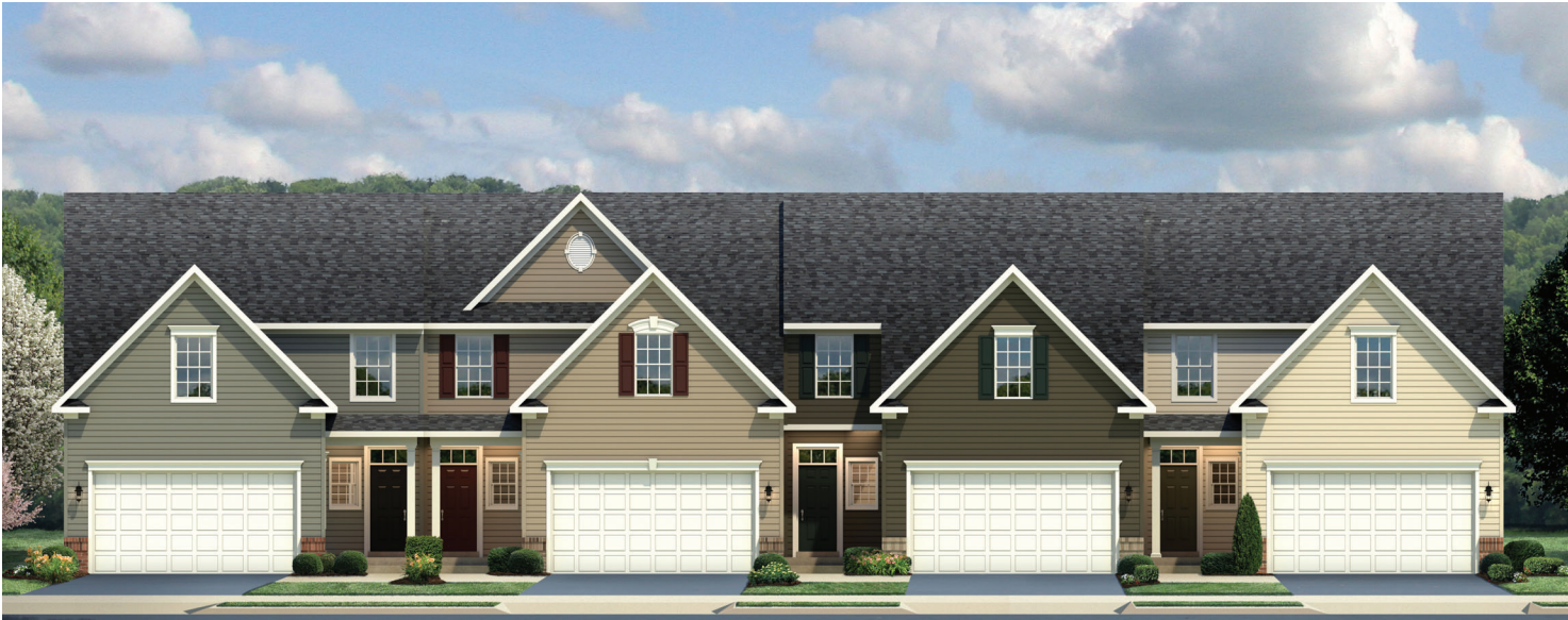
LEVEL ENTRY ON SLAB
